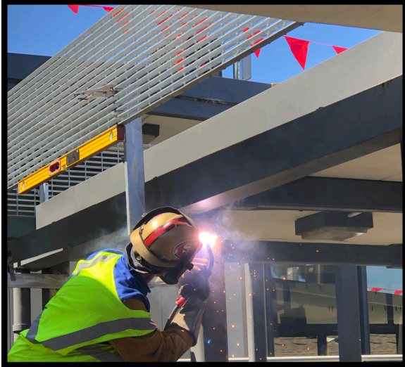
Pictured above - contractor installing grating panels at North ES
